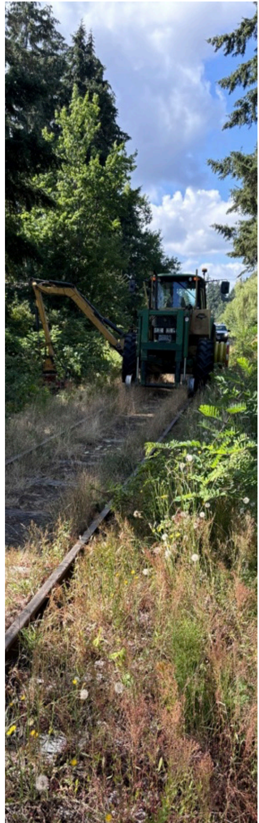
Victoria Subdivision – 2024 vegetation clearing in Nanaimo
