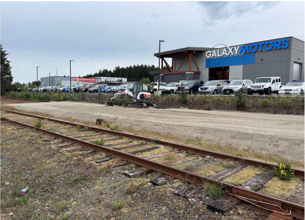
Work underway in Galaxy Motors Parking lot, Nanaimo
